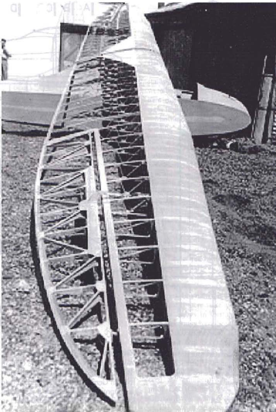
Top: Grunau Baby 3 D-5930 at Eisernhardt. Left: the original ESG31 'Stanavo'. Right: wing construction was difficult and expensive but good aerodynamically.
