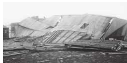
Above: London Gliding Club's hangar blown down in 1935. Below: LGC's original hangars before the 1935 storm, Falcon 1 in foreground.
