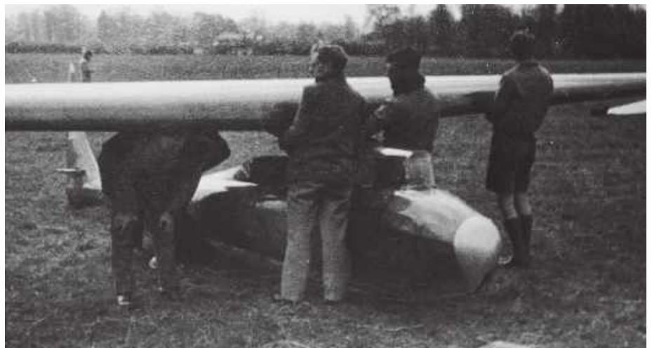
Above: connecting the ailerons? Below: lowering the wing on to the fuselage. Bottom: rigging wings on fuselage.
