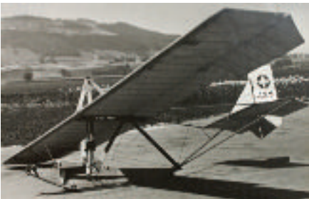
Above: the Karpf-Zögling (Swiss primary) HB-473 has a partly covered steel-tube fuselage. Below: the AeCS-Zögling (primary) HB-429 with a wooden fuselage. Is the number on the rudder correct? Swiss federal archives / Thomas Fessler Right: AeCS-Zögling HB-429 of Thomas Fessler in the museum of history at Grenchen in 2003. Thomas Fessler
