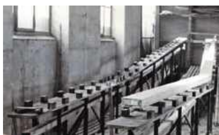
Above: working on the spar. Below: the spar jigs.
