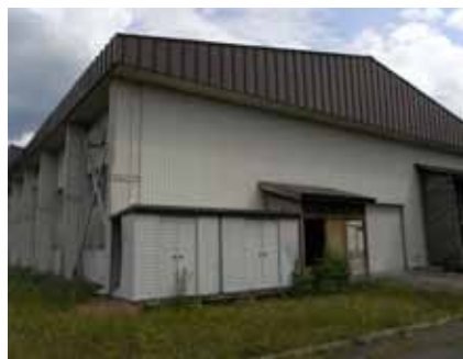
Old technical school building where the restoration work is carried out.
