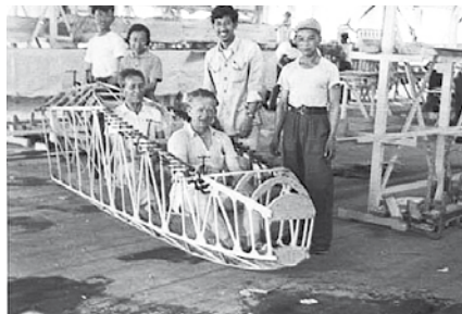
Jie Fang 1 fuselage under construction. Note Polish engineer in front seat.
