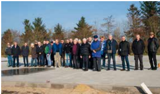
The concrete foundation gets load tested on 9 March 2014 following the DaSK AGM.
