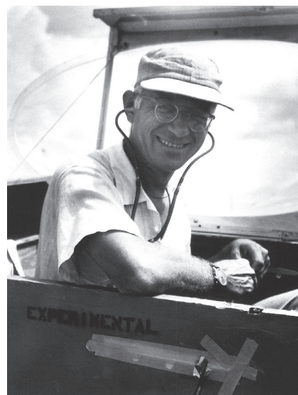
Dr. Raspet in the Test Engineer Position of a TG-3 with the stethoscope and probe for determining the transition from laminar to turbulent
