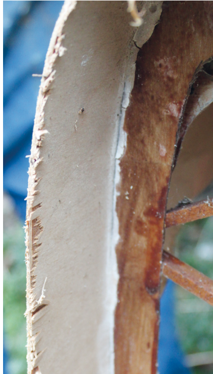
Close up of a nose-rib casein joint that has totally broken down on the 1935 prototype Kite 1.
