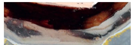
Aerodux is unmistakable with its characteristic dark purple/brown colouring. Here the glue has been freshly applied and readied for the plywood patch. Photo: Bruce Stephenson
