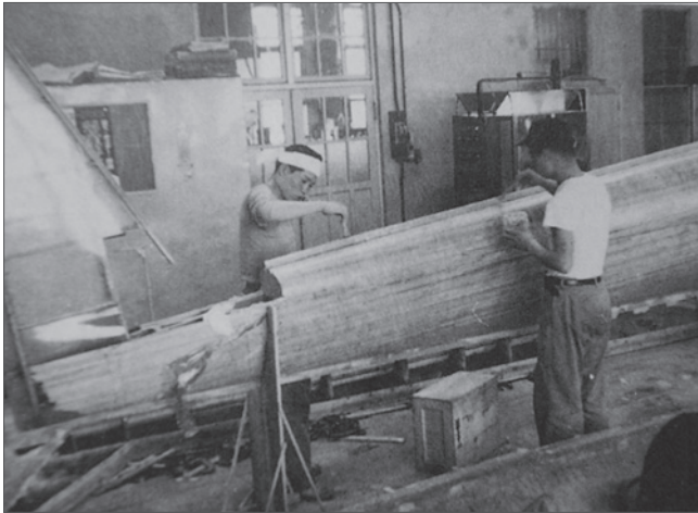
The LBS-3 under construction at Tokyo University
