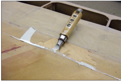
Expect the unexpected with deep inspections!
