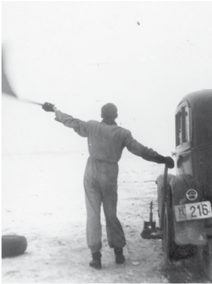
Waving a red flag, Alojz Petrin signals to the pilot of a sailplane climbing to release the car winch cable, which was mounted on the Ford Model A automobile owned by the 'Gull' group. From the registration plate we see that this was 216 th automobile registered in Banovina Hrvatska in 1940.
