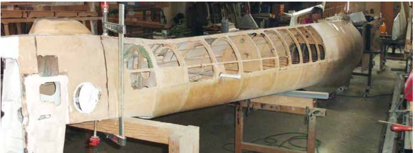
2013 saw the fuselage undergoing a deep inspection and repair of old unsightly repairs.
