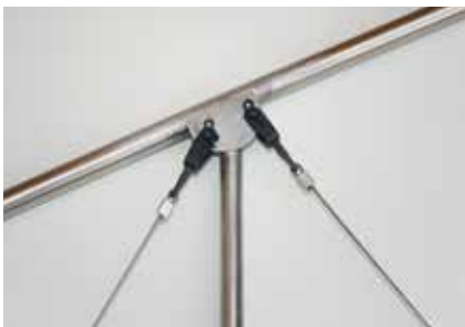
Some of the fittings now in place, all braced with 1mm control cable.
