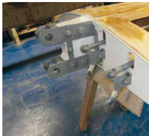
After cleaning and new paint, very slowly the reconstruction work could be started.
