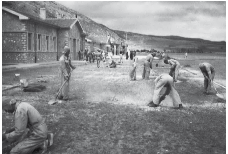
İnönü Gliding Centre under construction with men landscaping the camp. (Eskişehir)
