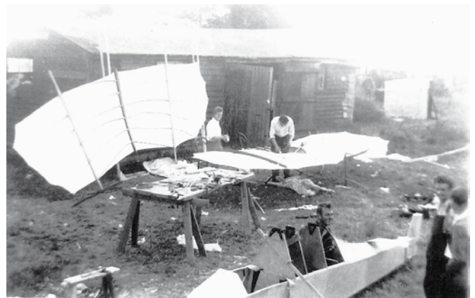
Another shot taken at right angles to the last of the same Lilienthal glider under construction, Luton Road. Note the Grunau Baby under construction in the foreground and the primitive conditions workers endured.
