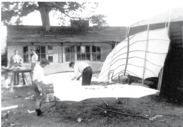
Construction of the Lilienthal glider at the workshops of Zander and Weyl on the Luton Road site
