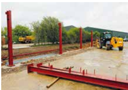
One big Meccano set...the steelwork arrives on site. Photo: Paul Haliday
