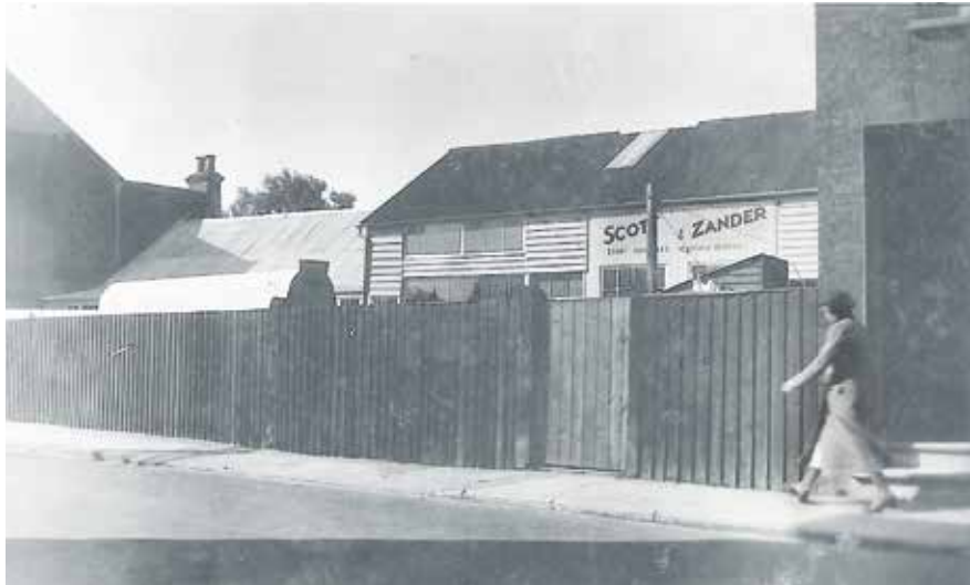
With a new business partner, the Scott and Zander factory opened its doors in 1937. In 1938 the company changed its name to Scott Aircraft and moved to smart modern buildings here on Mathew Street.
