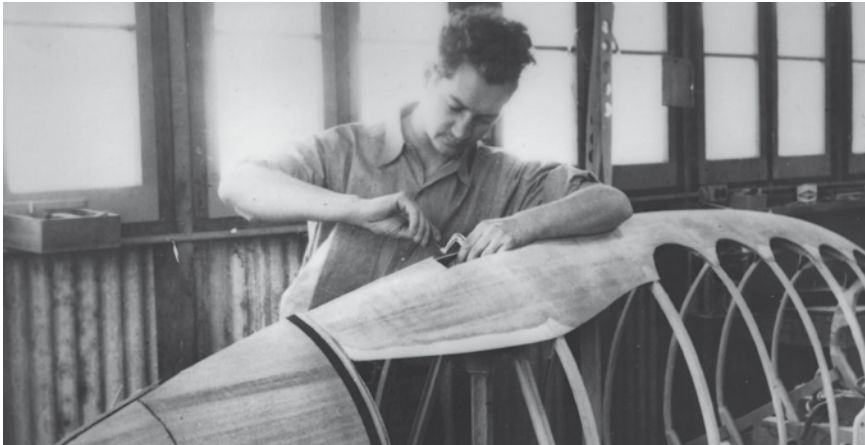
Harold Huber skinning his #3 scarfed pod prototype. He did not complete it until Dec. 1939 and thus received s/n 114. Photo: Jim Campion
