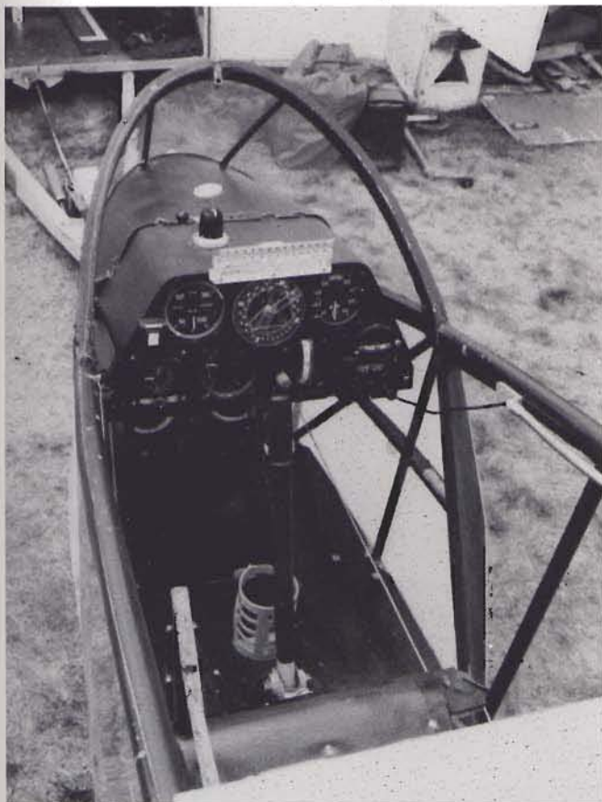
High speed panel in Ernst Walter's Mü 13d. Photo C.Wills.
