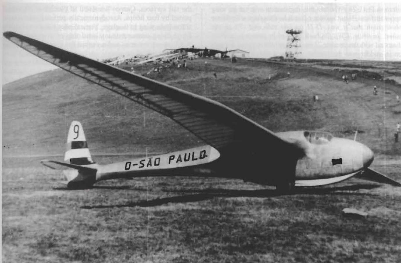
The Fafnir II at the Wasserkuppe which was built in 6 weeks, and just before its record breaking, first soaring flight, which ended in Czechoslovakia.
