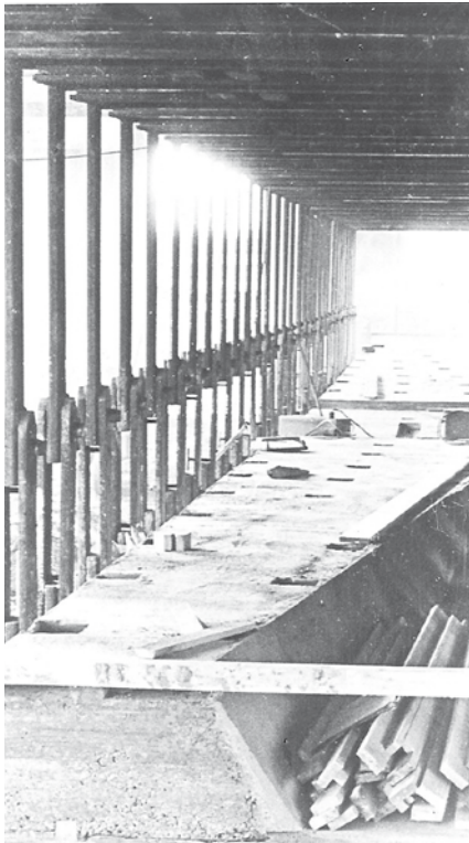
Constructing the 25m press Photo G. Remy
